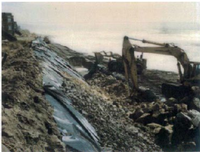
Photograph 1: Pajaro Dunes North Rip-rap Revetment Under Construction in 1983
