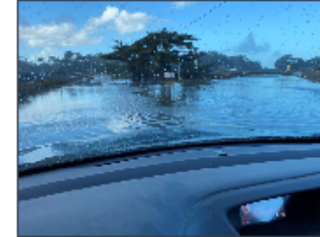
High water levels cause flooding of low elevation infrastructure (road crossings)
