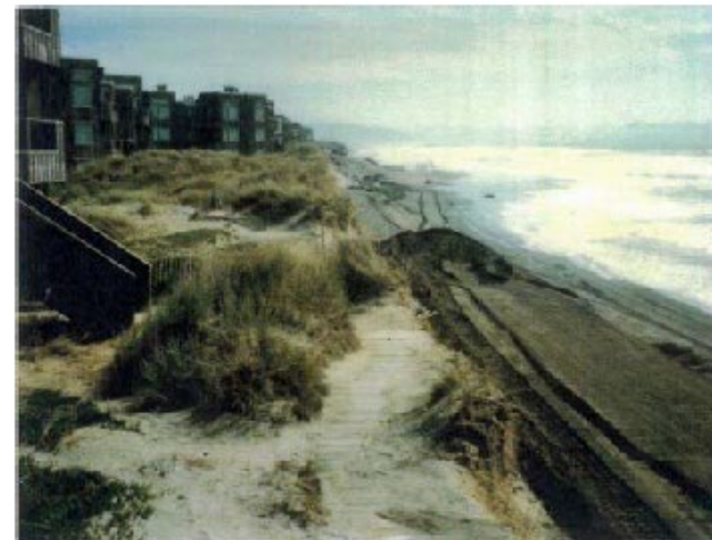
Photograph 3: Pajaro Dunes North Rip-rap Revetment Under Construction in 1983
