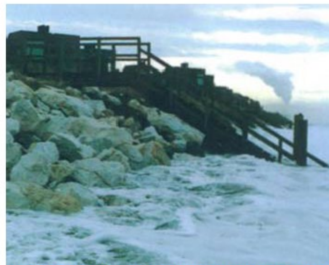
Photograph 4: Pajaro Dunes North Rip-rap Revetment and Stairway Under Wave Impact after Construction in 1983
