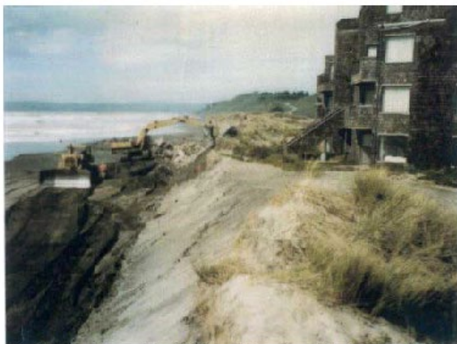
Photograph 2: Pajaro Dunes North Rip-rap Revetment Under Construction in 1983
