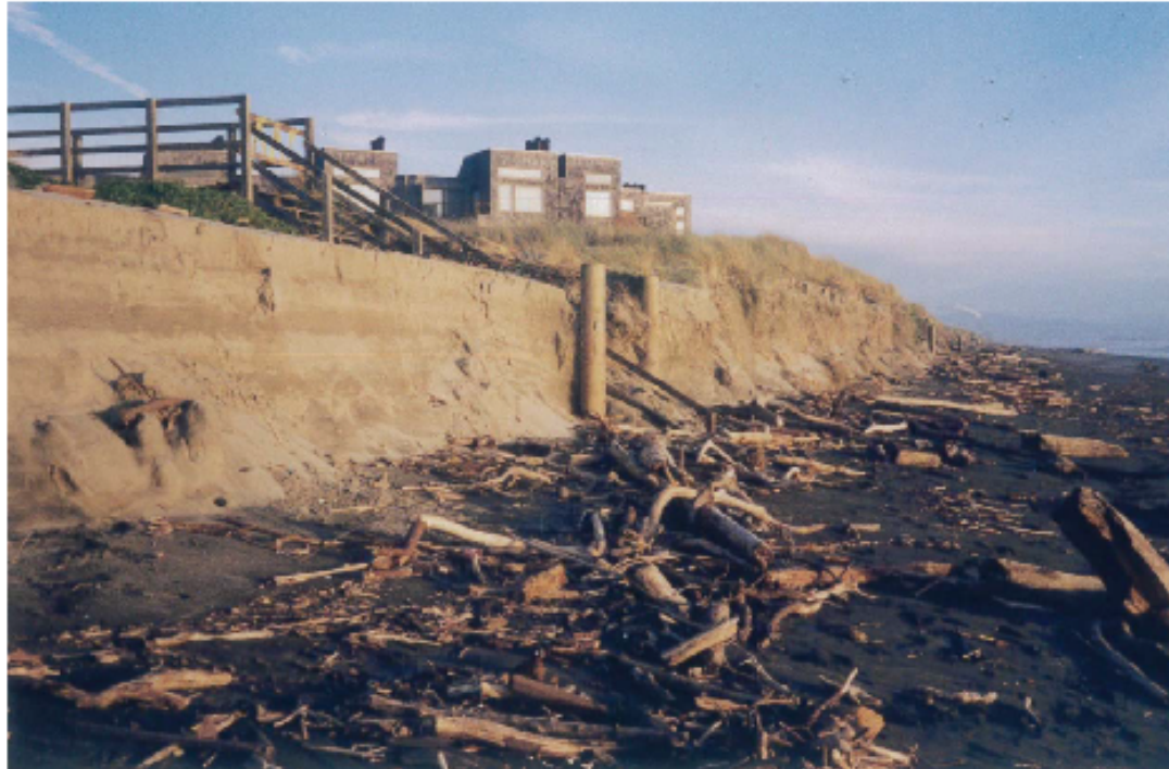
Photograph 6: February 12, 1998 Photograph at Building H Stairway
