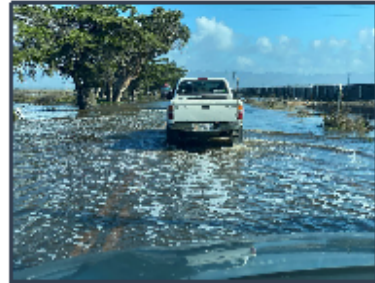
Flooding of low elevation infrastructure (road crossings) causes safety problems
