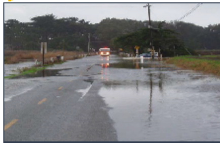
Flooding causes problems for emergency and public access
