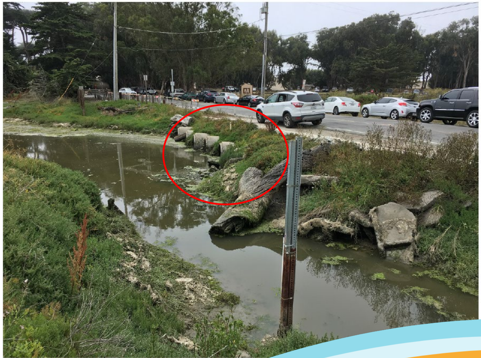
Figure 9. Beach Road Crossing at Watsonville Slough – view of
